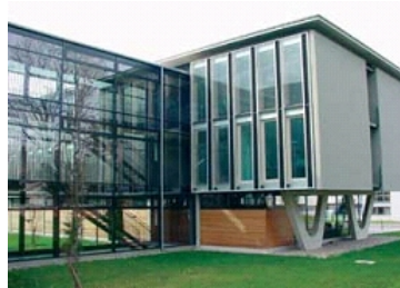
New office building of Badenova in Offenburg, GER
